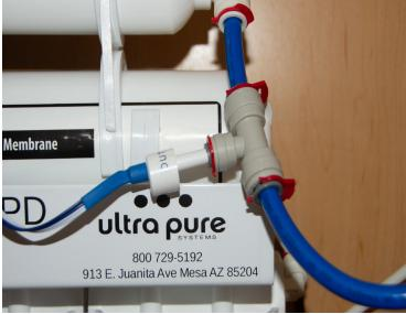
Once all the steps above are complete you are ready to turn on the Angle ball valve # 2 that was installed onto the city water ball valve and tank ball valve that was screwed on step 6.
